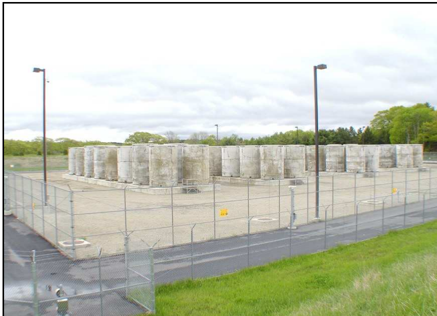
Figure 14. Dry Cask Storage Facility at the Decommissioned Maine Yankee Reactor Site (source: http://www.maine Yankee.com )
